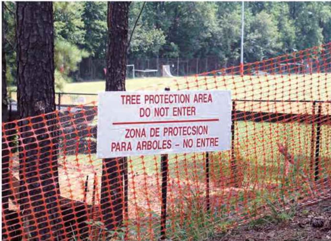
Figure 6.05a Tree protection zone. A protected zone preserves roots and soil and keeps branches clear of contact with construction equipment and materials.
